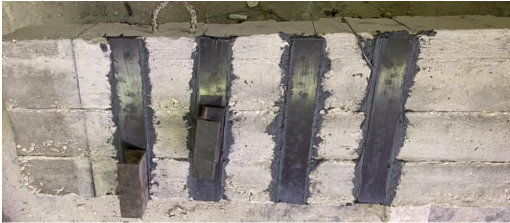
Fig (4): Beam During CFRP Strengthening
